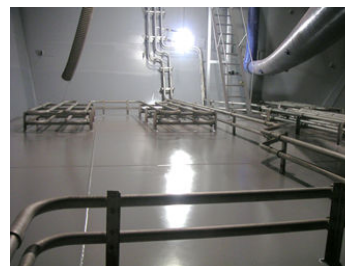
Completion of application by Phenol epoxy coating
