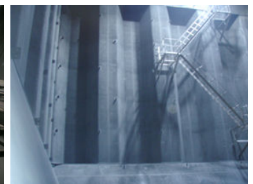
Completion of application by Inorganic zinc coating
