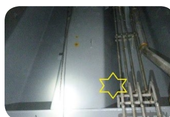
Tank Coating Tested with Butterworth Method
